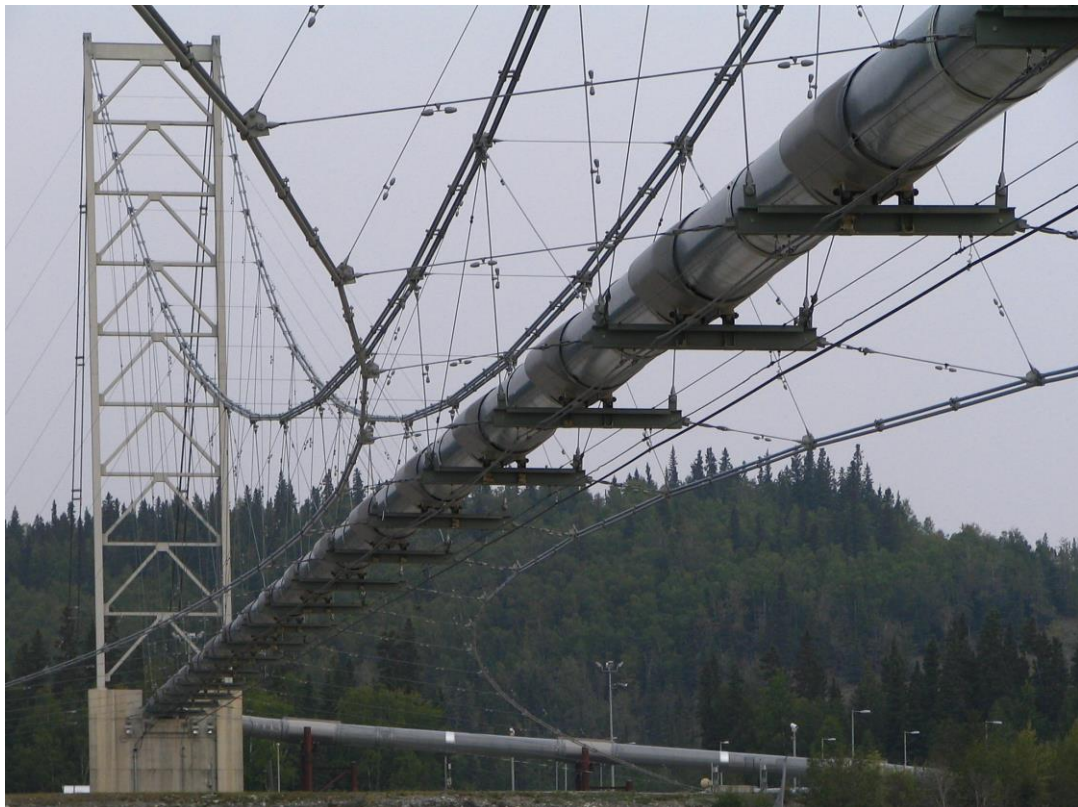
Alyeska Pipeline. Bridge designed by Prof. NEWMARK over Tanana River, 1977.
