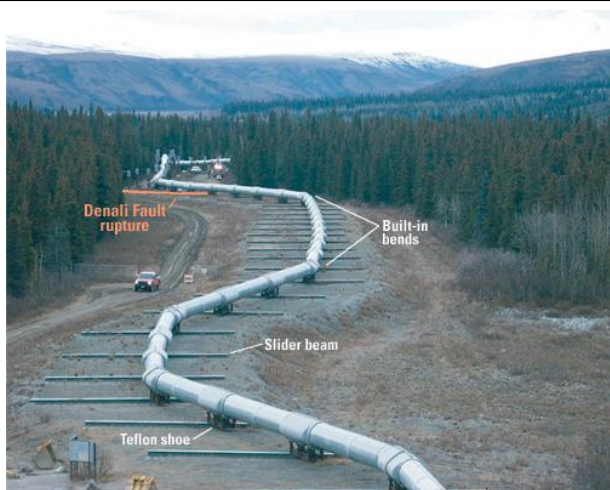
Alyeska Pipeline. Anti-seismic design of pipeline.
