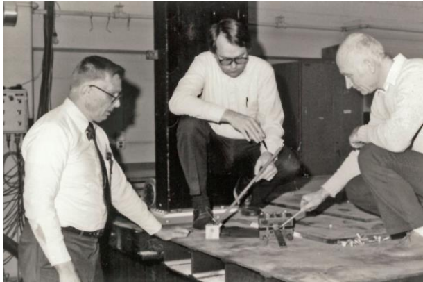
Graduate students Steve McCabe and Dave Segal, and W. J. Hall, Professor and Head of Department, discussing fabrication of a steel model structure to be tested on the departmental earthquake simulator.
